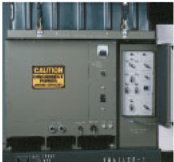
EALS Regulator and Primary Control Panel
